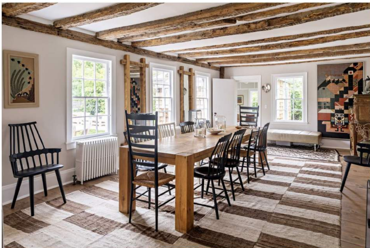
Stephen Harvey and Perry Sayles removed dropped ceilings in their 1788 farmhouse, revealing hand-hewn beams. DOROTHY HONG FOR THE WALL STREET JOURNAL
